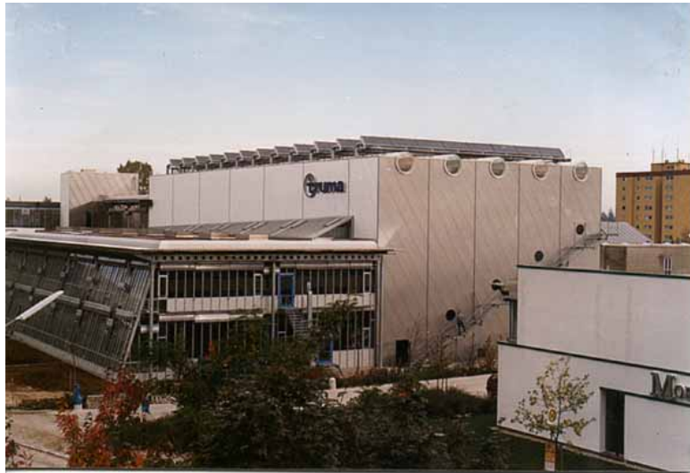
Hochregallager, Truma Putzbrunn, 210 m 2
